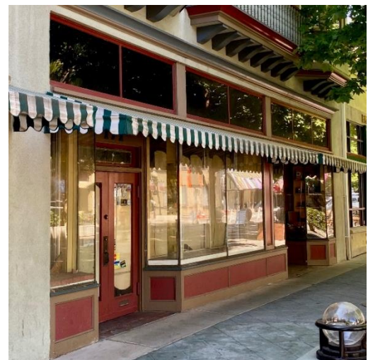
Fig. H.10: Entry alcove at street-facing building facade.
