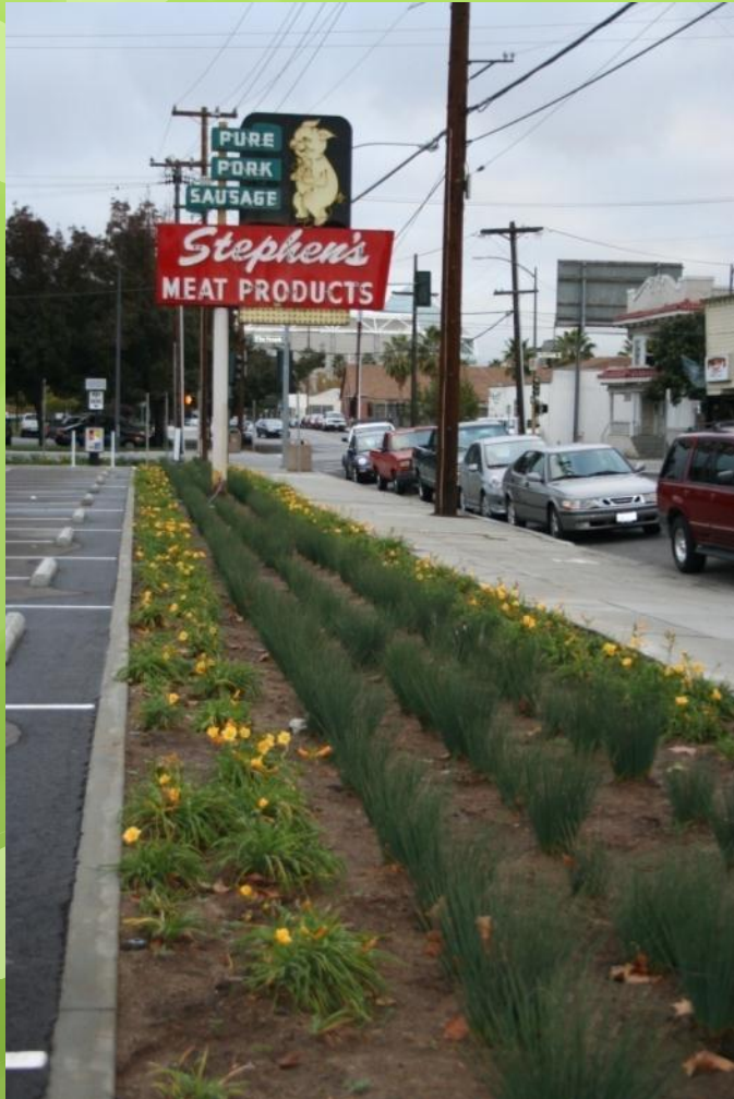
Bioswale adjacent to parking lot near Diridon CalTrain Station in San Jose
