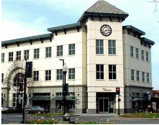
Fig. H.26: Building roof forms fronting Castro Street should reinforce the character of the historic commercial buildings with flat roof forms, parapets, cornices and decorative details.
