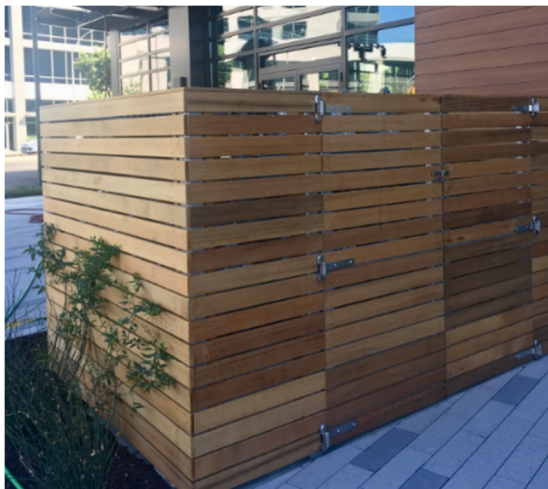
Fig. H.20: Service facilities should be screened with enclosures and devices consistent with the building architecture.
