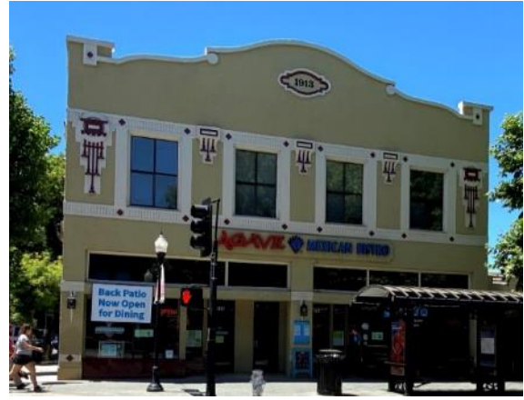
Fig. H.26: Building roof forms fronting Castro Street should reinforce the character of the historic commercial buildings with flat roof forms, parapets, cornices and decorative details.
