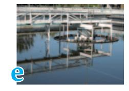
The water clarifies as the microorganisms fall to the bottom of the **settling basins**. The settled organisms are pumped to the blend tank or the aeration basins for reuse.
