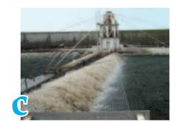
The water trickles through two-story towers called fixed film reactors. Inside the towers, microorganisms, forming a film on a plastic honeycomb, eat the organic matter in the wastewater.
