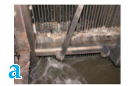
The treatment process begins as raw wastewater passes through a bar screen to remove roots, rags, plastic, and other large
