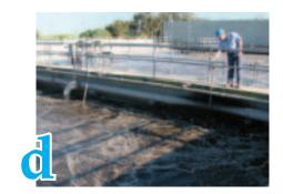
Air bubbles up through the wastewater in aeration basins like giant aquariums. The air supports microorganisms that remove the remaining dissolved solids and ammonia, a chemical toxic to fish.
