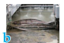
The wastewater is pumped into sedimentation tanks, where floating material such as hair and grease are skimmed off. The thick sludge settles to the bottom. Both the sludge and floating material are pumped to blend tanks for processing.
